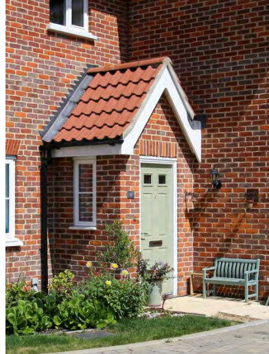
Composite door with brick porch
