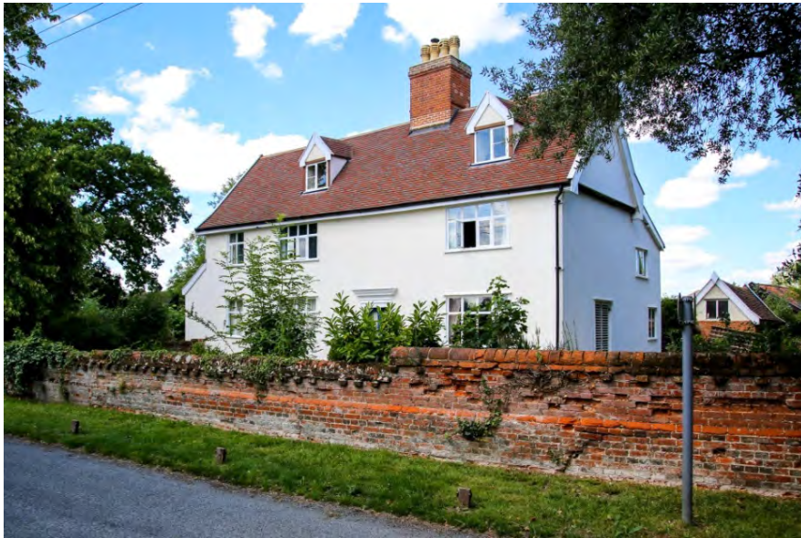
Brick wall, College Farm House
