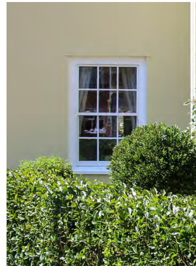
White sash window with glazing bars
