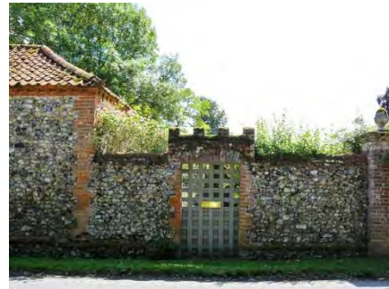
Flint wall, Barningham House
