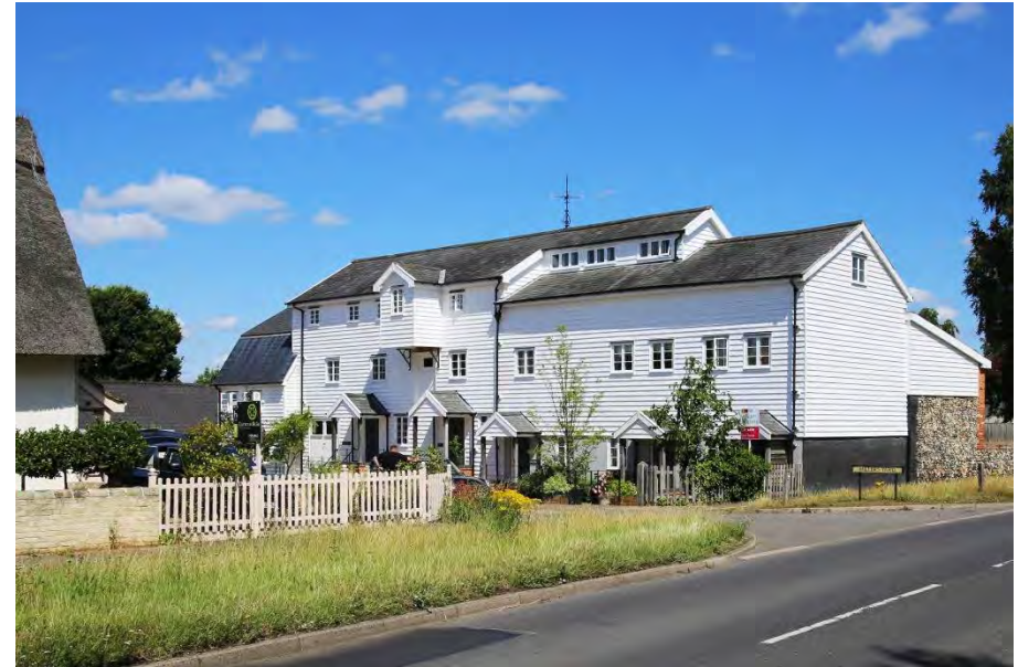
Former Steam Mill
