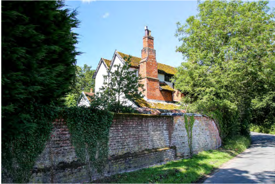
Brick chimney stacks of Old Hall
