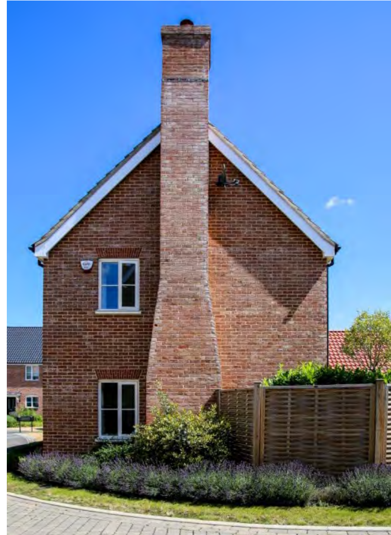
Example of the brick chimney stack implemented in the recent development on Linwood Close.
